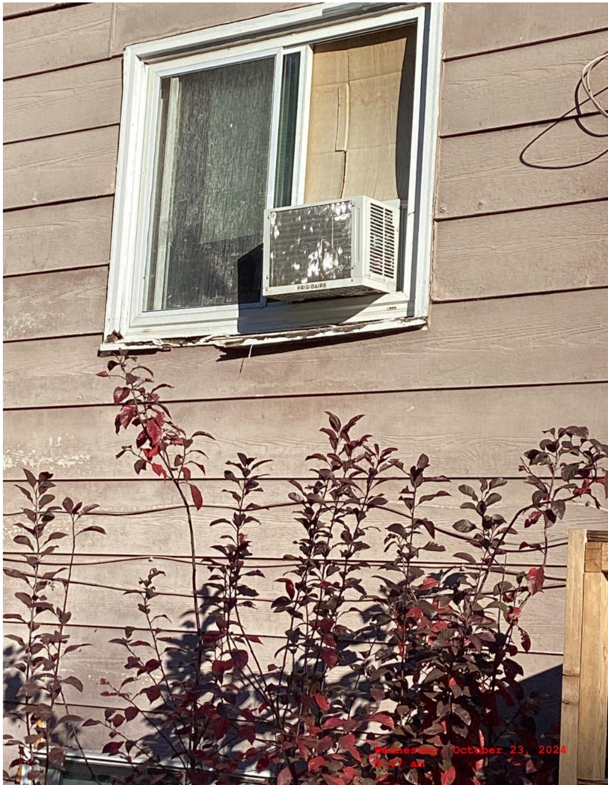
EXHIBIT C3: UPPER FLOOR SOUTH WINDOW DAMAGE
