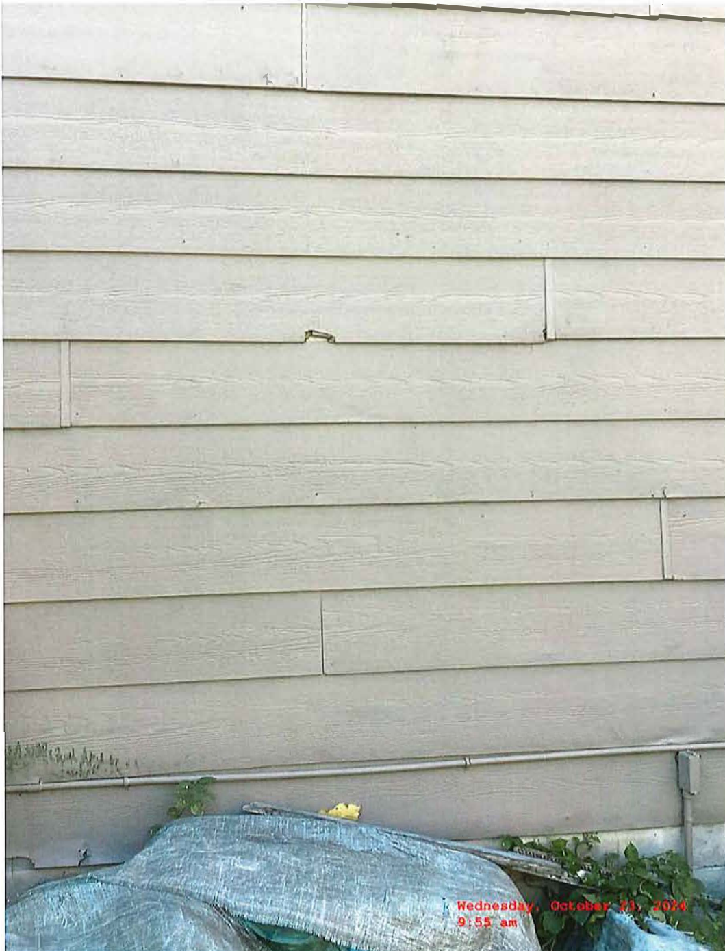
EXHIBIT C8: NORTH SIDE OF DWELLING-HOLES IN SIDING, MISSING SIDING JOINT SPLICES
