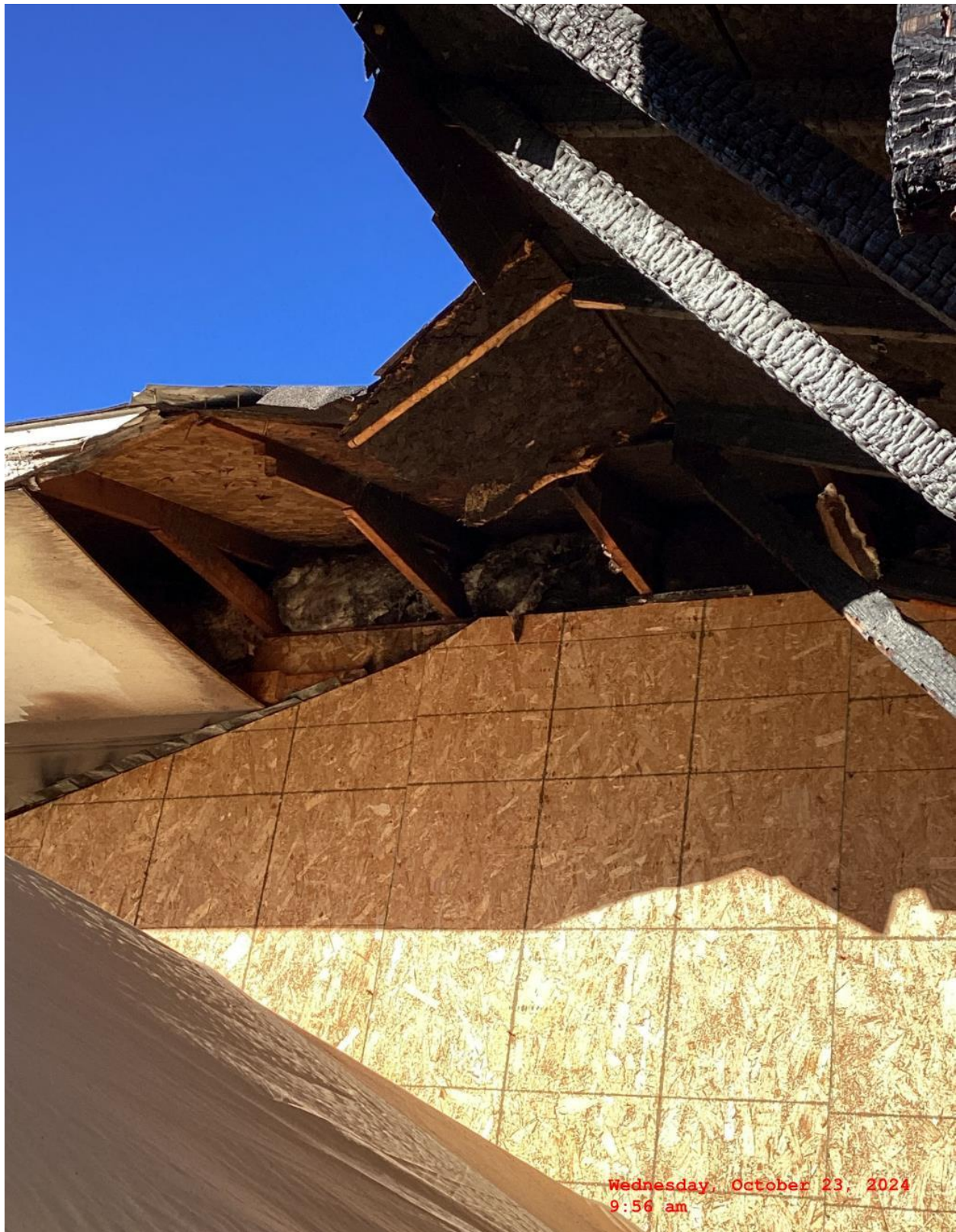
EXHIBIT A3: FIRE DAMAGE AT FORMER ATTACHED GARAGE-EAST SIDE OF DWELLING
