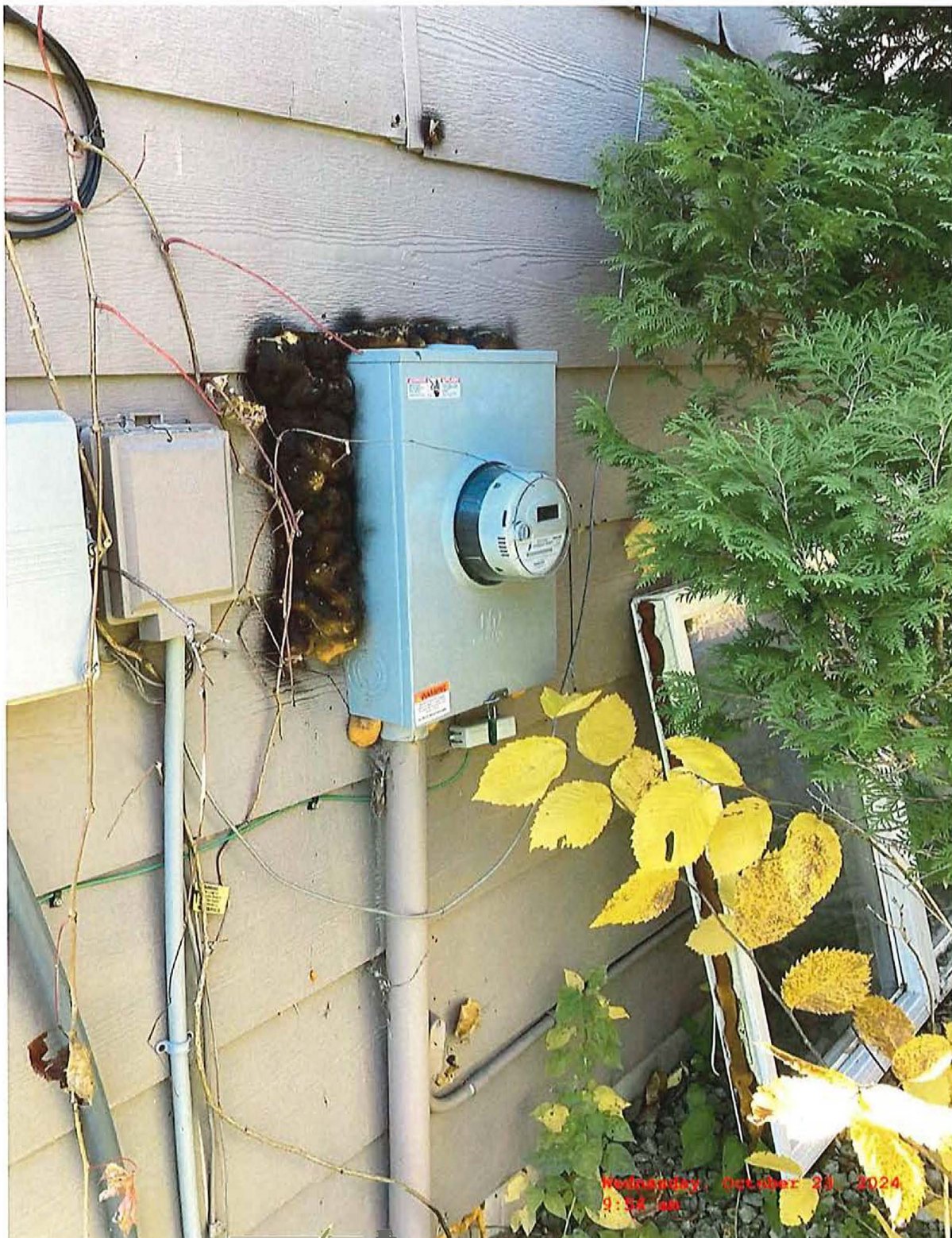
EXHIBIT C7: ELECTRICAL METER PANEL ON NORTH SIDE OF DWELLING-INADEQUATE SEALING AROUND BOX-MOISTURE ISSUE AT SIDING
